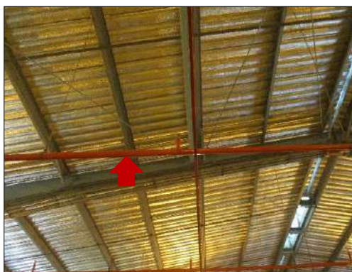
Water Deluge System / Water Spray System
